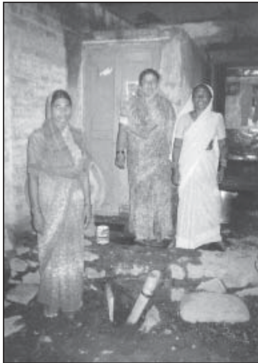
Women of Rajuri outside the toilet facilities they constructed.
